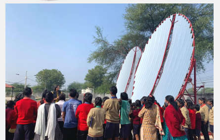
SOLAR COOKER INSTALLATION
